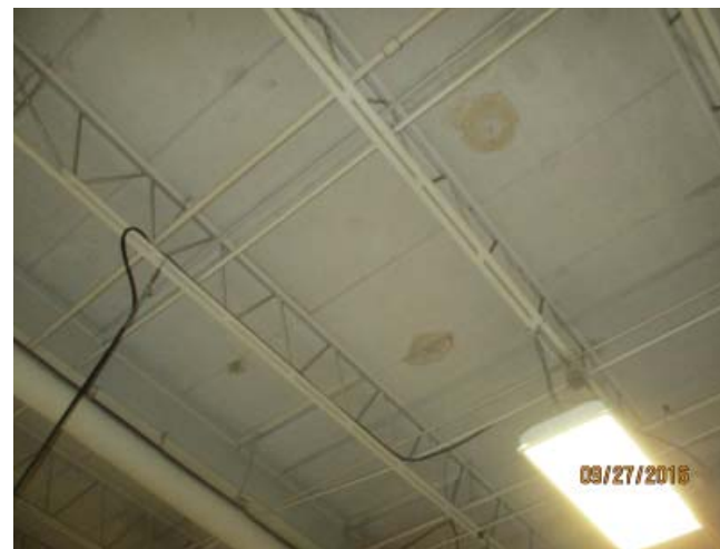
Tectum deck with tie down connections
