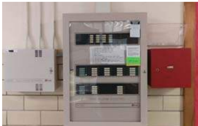
Fire alarm control panel
