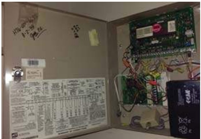
Security alarm control panel
