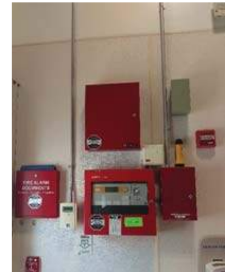
Fire alarm control panel and Wireless master box
