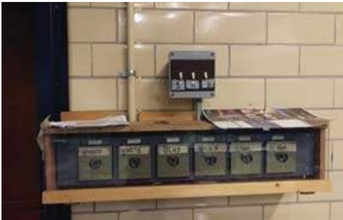
Dimmers for controlling performance lights
