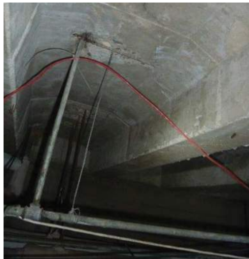
Spalling concrete
