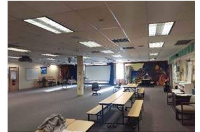
Recessed Parabolic Fixtures in CBHS Assembly Area
