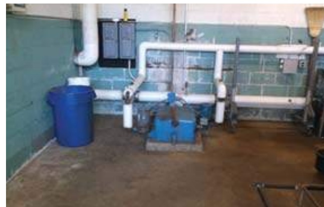
Condensate Pump Unit
