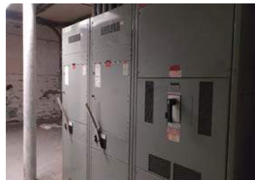
Service Disconnect Switches
