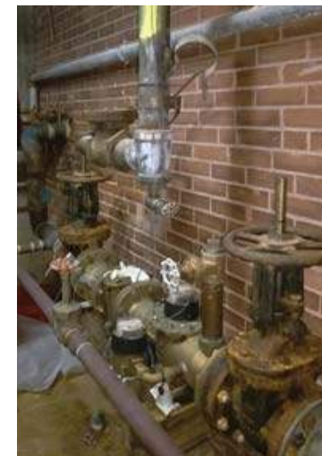
Domestic Water Entrance with No Grounding Electrode Connection
