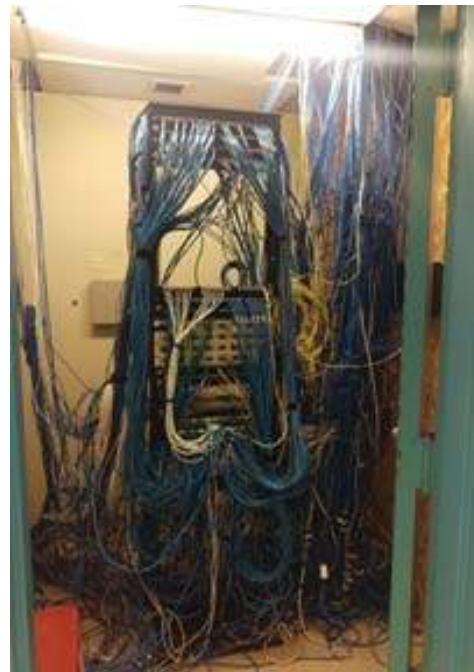
An IDF Where old data cable were abandoned when an update was completed.
