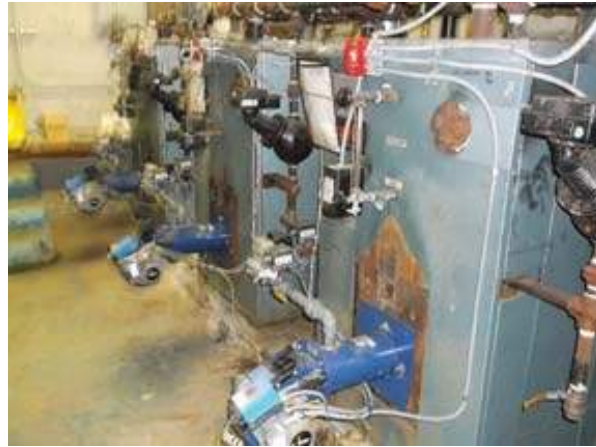
Gas Converted Boiler Plant
