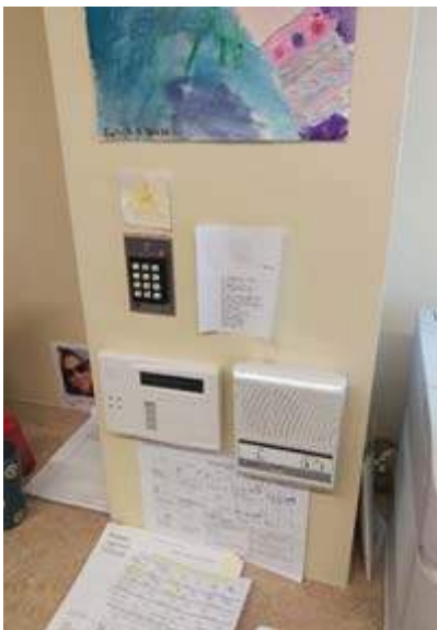
Main Office Entry Intercom and Access Control and Intrusion Alarm Keypads
