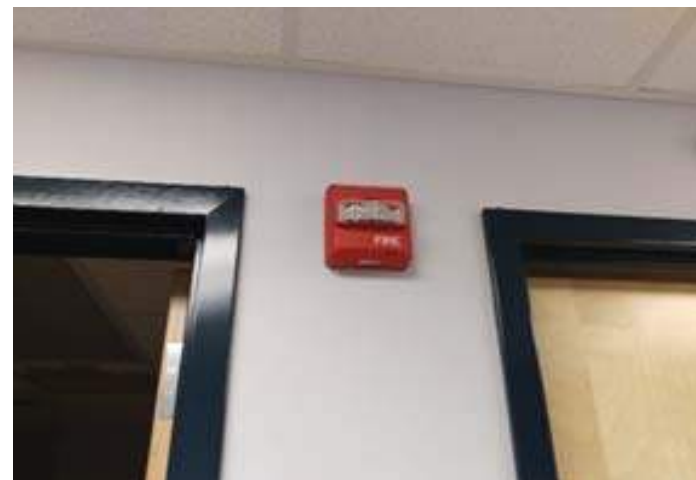
A modern notification appliance in the Health Center
