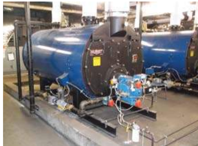
Recently Installed Firetube Boiler Plant
