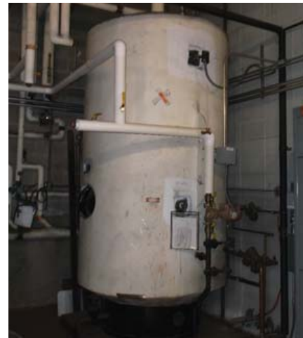
Indirect DHW Tank – Original Vintage
