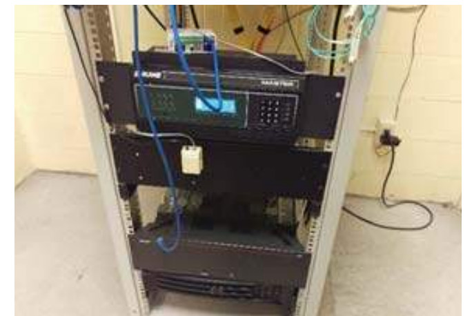
Master clock and paging amplifier
