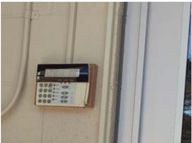
Intrusion Detection Keypad in Main Entrance Vestibule
