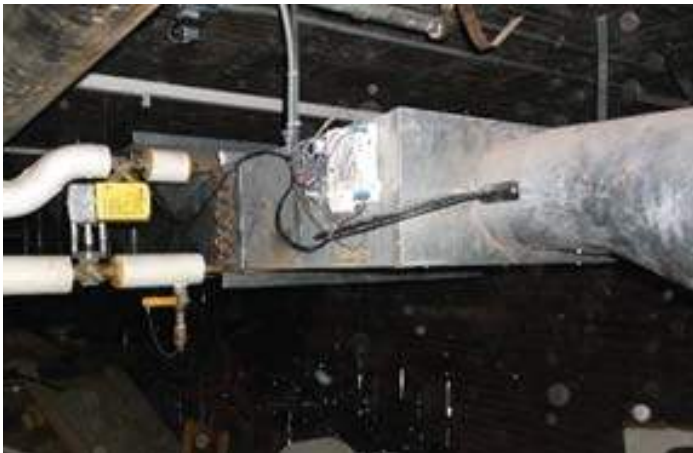
Indoor H&V Unit with New Actuator
