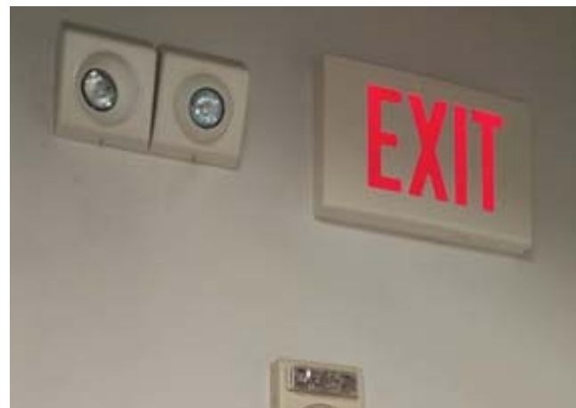
An Exit Sign and Emergency Light Heads
