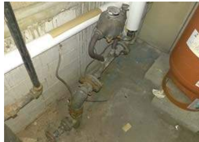
Grounding electrode connection at water main has been cut off.
