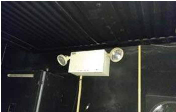
Typical Emergency Lighting Battery Unit
