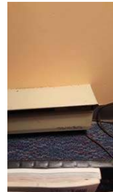
Electrical cords routed near baseboard heater
