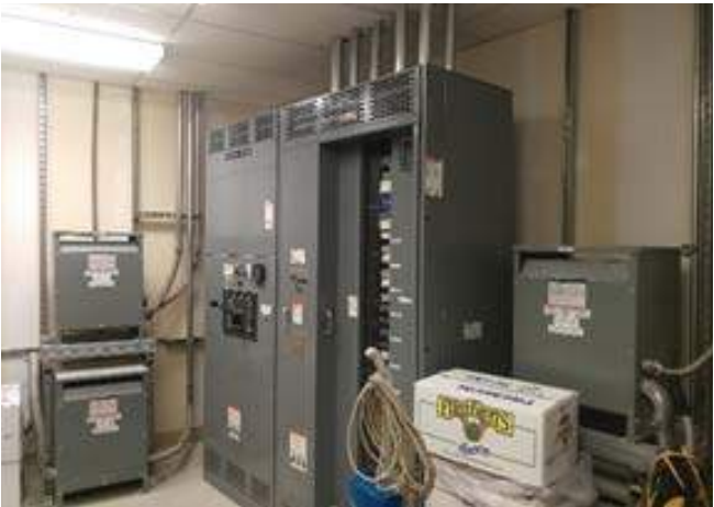
Main distribution switchboard
