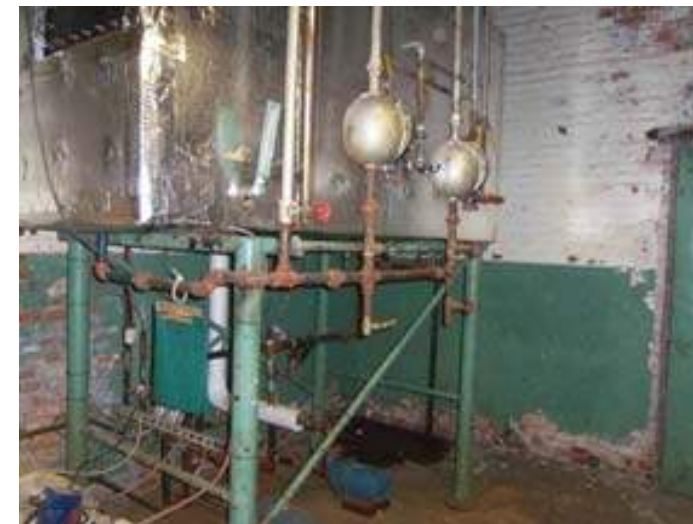
Boiler Feed Pump System
