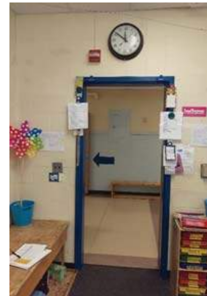
Typical classroom fire alarm strobe
