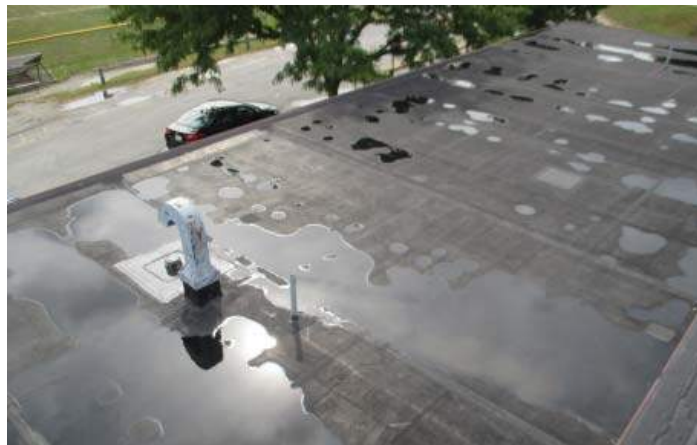
Poor roof drainage at low roof near MPR
