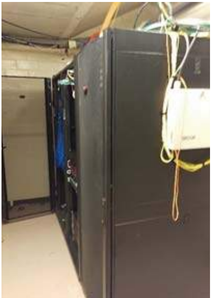
MDF and network core equipment in enclosed cabinets in data center.
