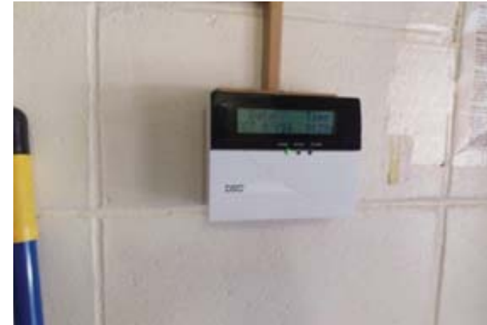
Intrusion Alarm Keypad
