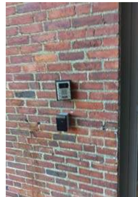
Video intercom and card access at entrance near 1983 addition.
