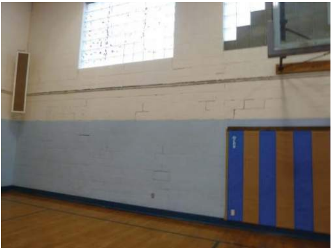
Stepped cracks
