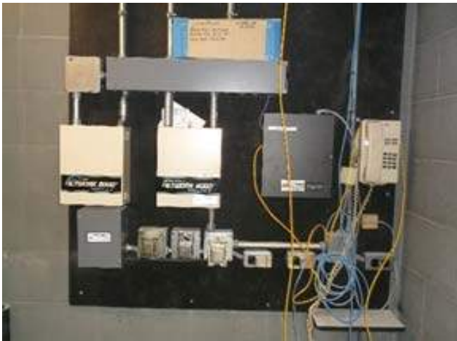
Vintage Pneumatic Temperature Control Panel
