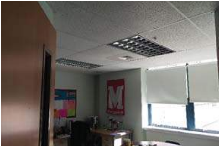
Parabolic fixtures in administration areas
