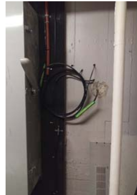
Fiber Optic and CATV entrance cables
