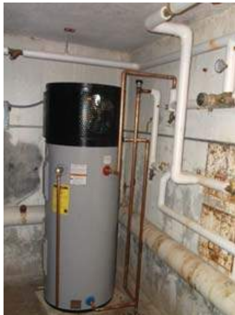
New Heat Pump Water Heater
