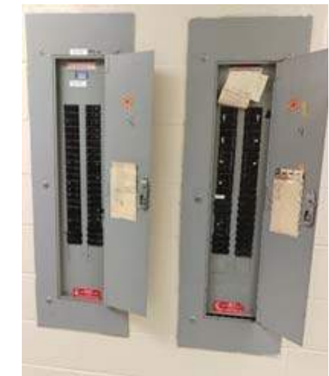
Typical 1983 vintage branch-circuit panelboards
