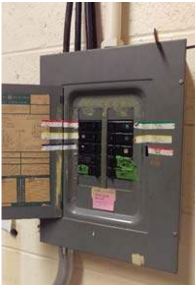
Old load center on stage
