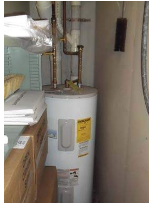
Missing pipe insulation at water heater
