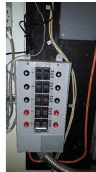
Generator transfer device
