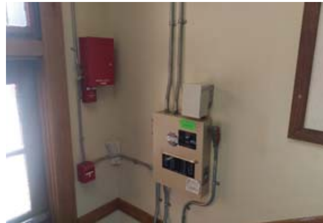
Fire Alarm Control Panel
