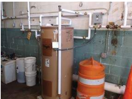
Electric Water Heater &amp; Mixing Valve
