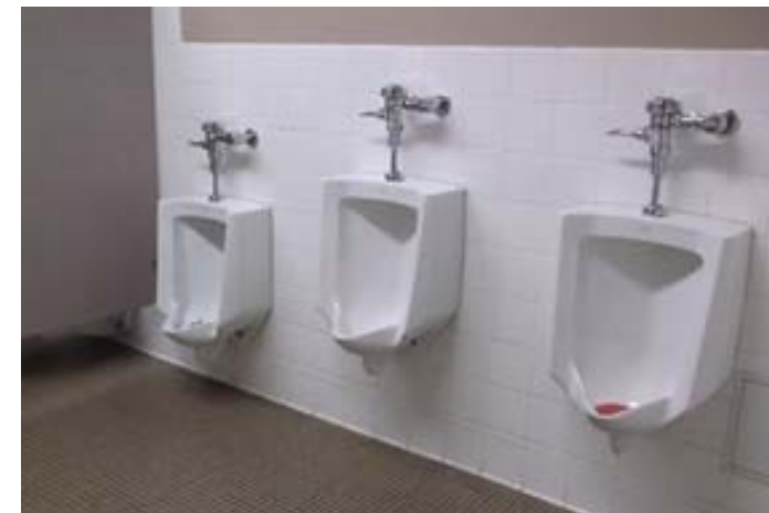
Recently Replaced Urinals & Flush Valves
