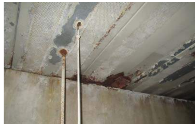
Second floor deck corrosion below bay doors
