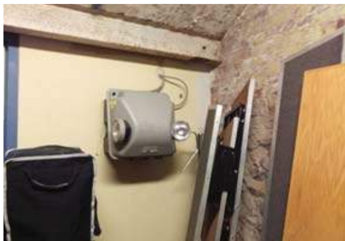
Newer emergency lighting unit in electric room
