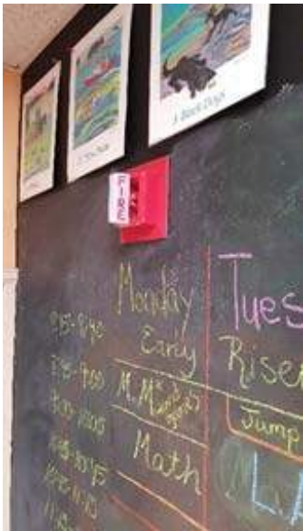
Fire alarm horn/strobe
