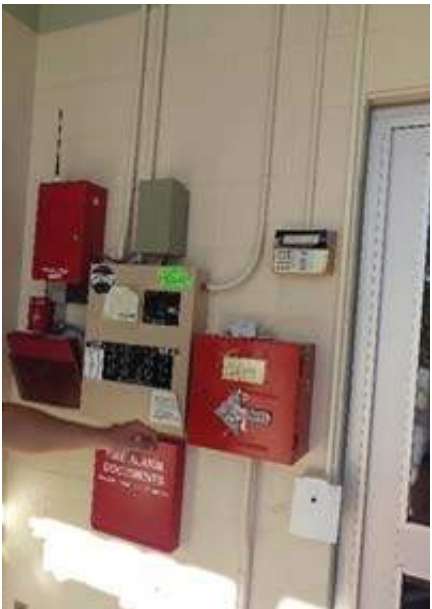
Fire Alarm Control Panel
