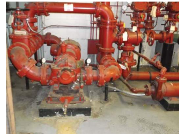
Fire Sprinkler Entrance With Pump
