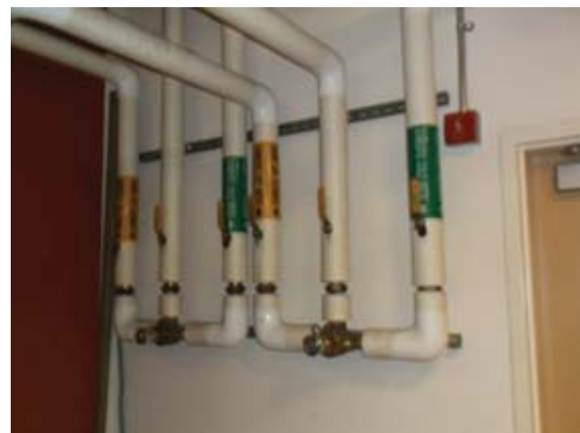
DHW Tempering Valves
