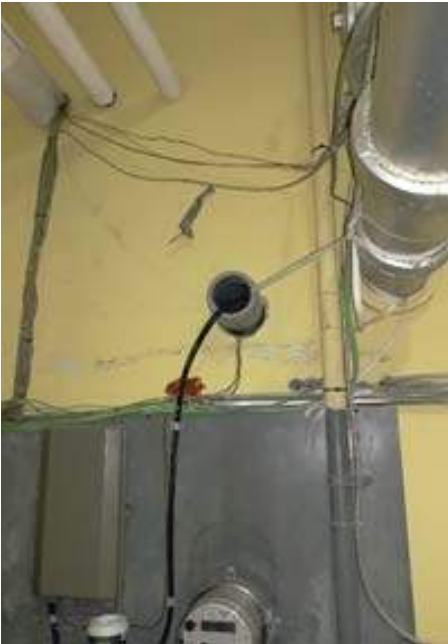
Telephone utility demarcation point
