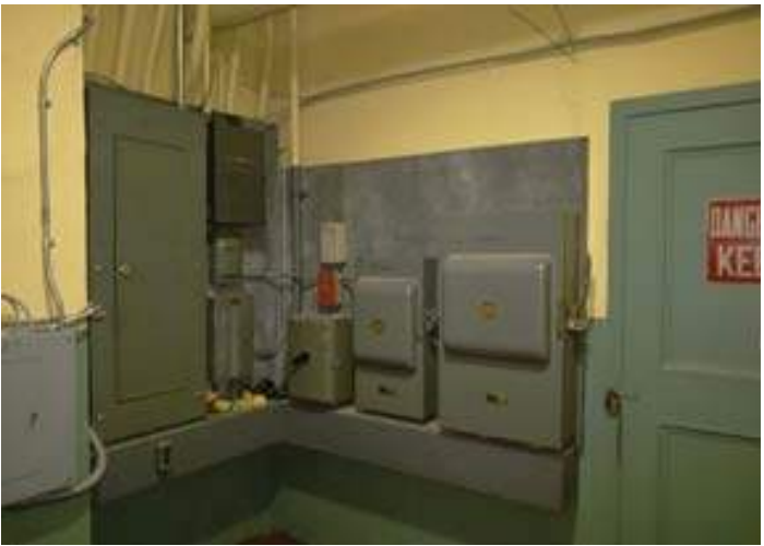
Service disconnect switches
