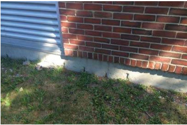
Spalling at foundation
