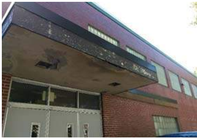
Old incandescent fixtures at a secondary entrance canopy
