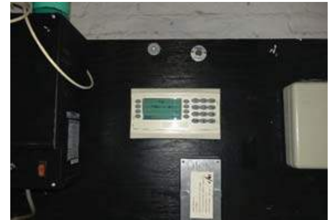
Intrusion Alarm System Keypad
