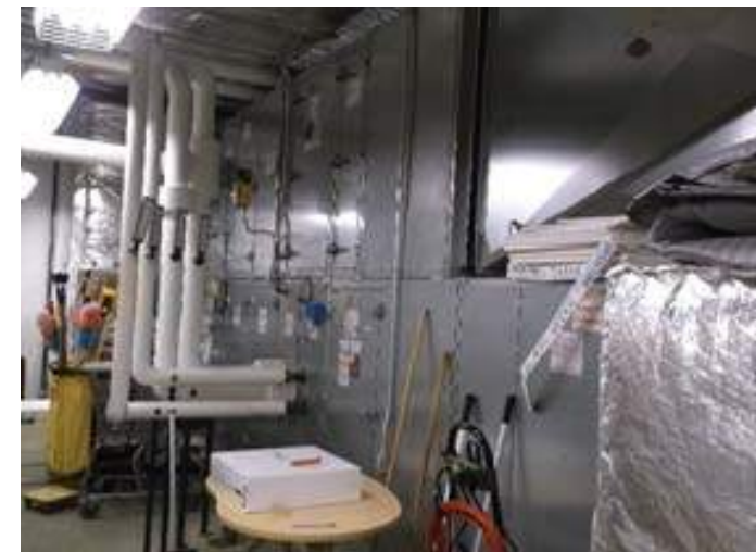
Air Handler with Heating & Cooling
