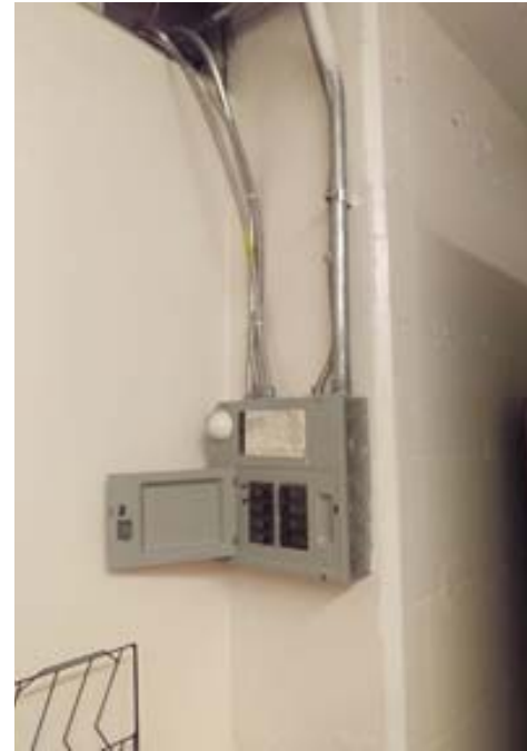
Small load center in 3rd floor work room
