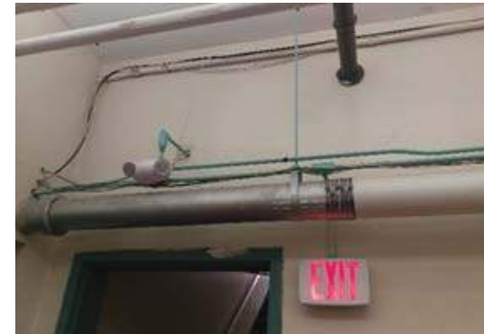
An LED emergency light and exit sign
