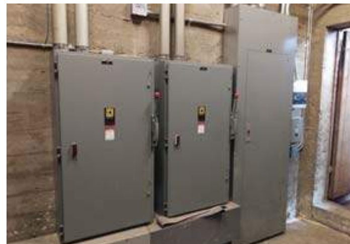
Service disconnect switches and MDP
