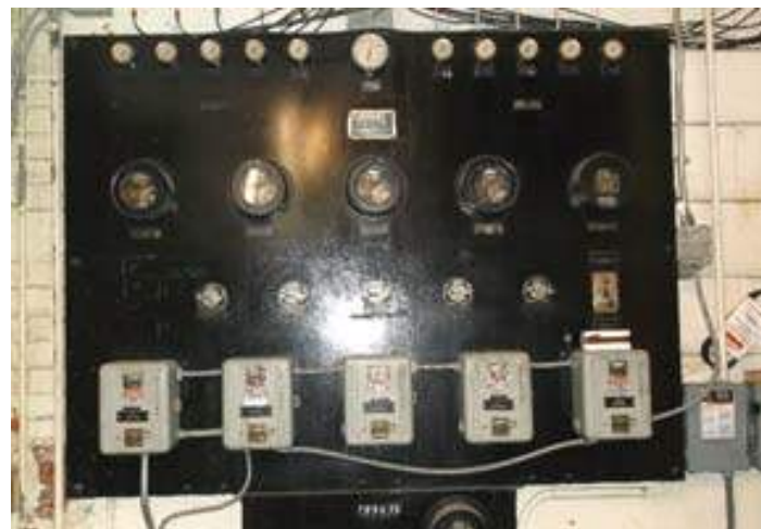
Vintage Pneumatic Temperature Control Panel
