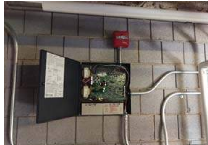
A Notification Power Supply with Old Batteries in a Mechanical Penthouse
