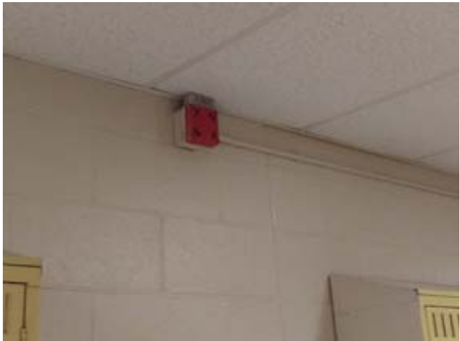
An obsolete notification appliance
