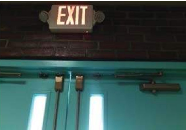
An LED Combination Exit/Emergency Light
