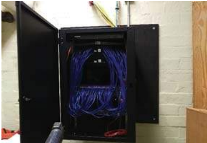
IDF #5 – typical enclosed IDF cabinet
