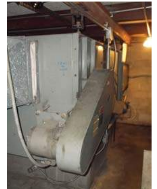
H&amp;V Air Handler in Gym Mezzanine
