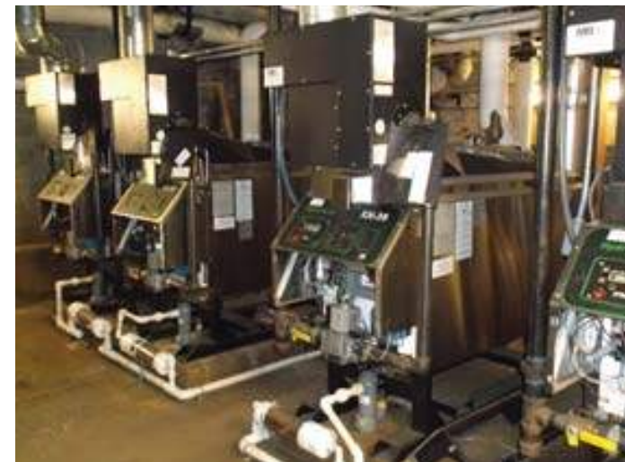
Condensing Boiler Plant
