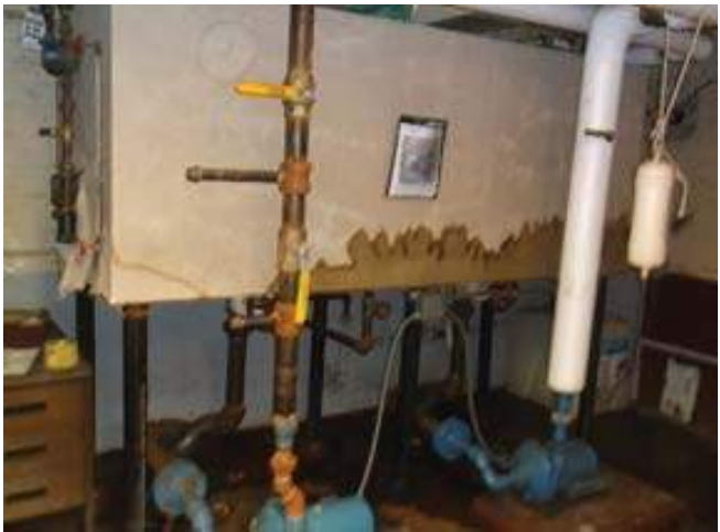
Vintage Boiler Feed Pump Unit
