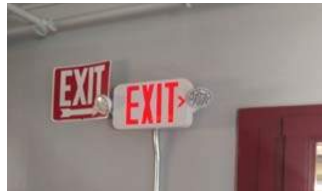
Combination Exit/emergency light with LED heads.
