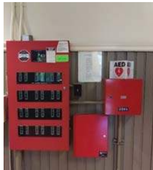
Fire alarm control panel
