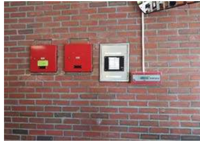
Current Fire Alarm Annunciator and an Abandoned Adjacent Annunciator
