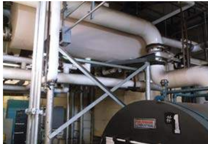
Steam to HW Heat Exchanger
