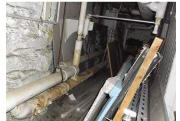
Vintage Steam Piping Insulated and None
