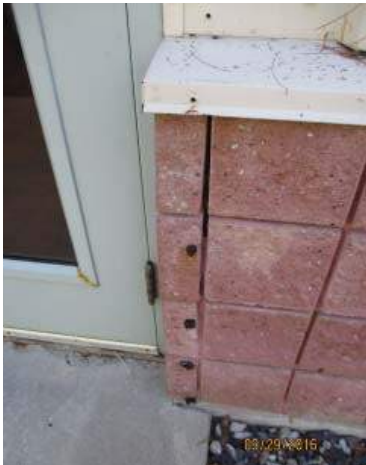
Open masonry joints
