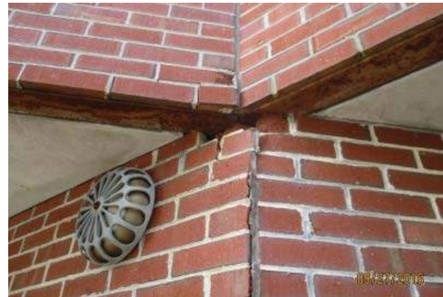
Corroding relieving angle
