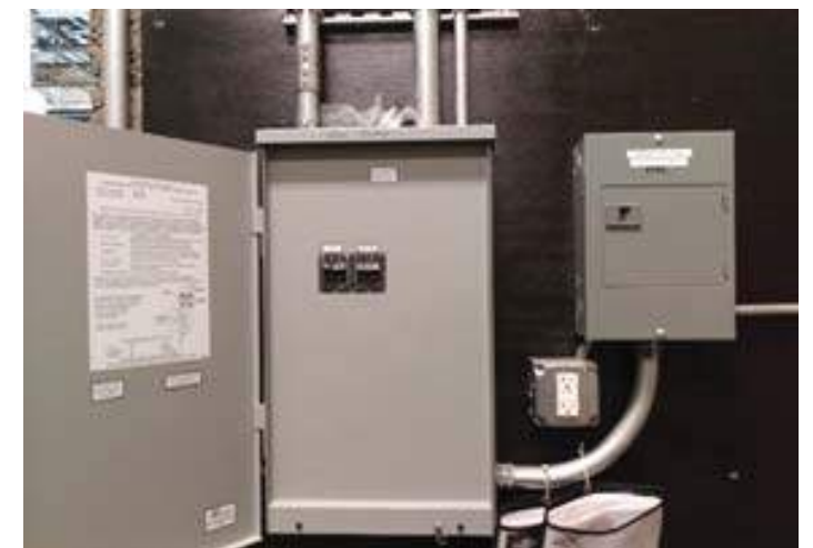
Automatic transfer switch and generator-backed load center
