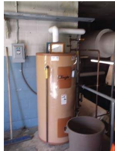
40 Gal Electric Water Heater
