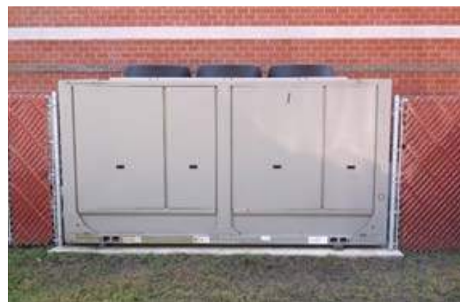
Cooling Plant—Air Cooled Chiller
