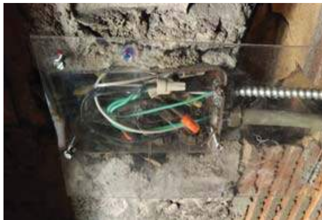
Junction box in attic containing old cloth-covered wiring as well as modern wiring.
