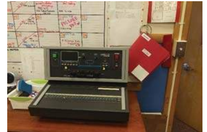
Intercom System Head End
