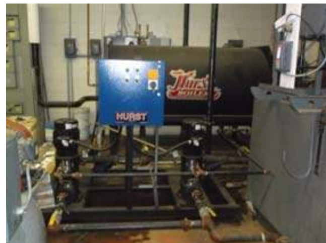
Boiler Feed System
