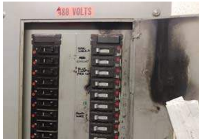
An Old Panelboard that Once Experienced a Fault
