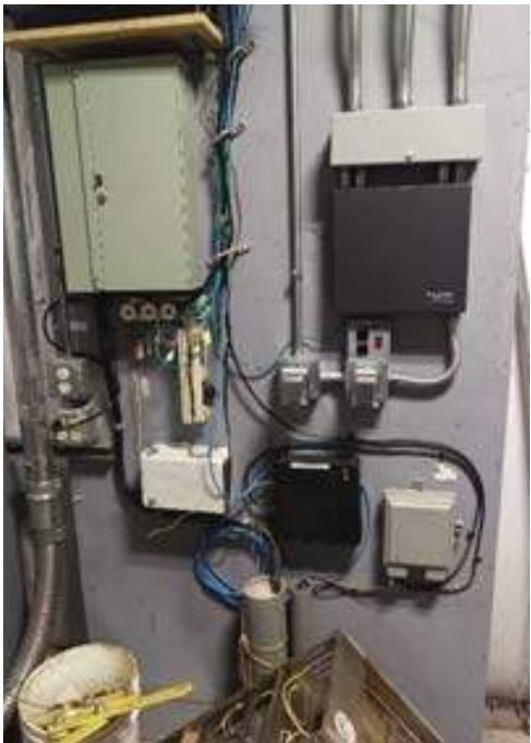
Telephone and CATV demarcation point
