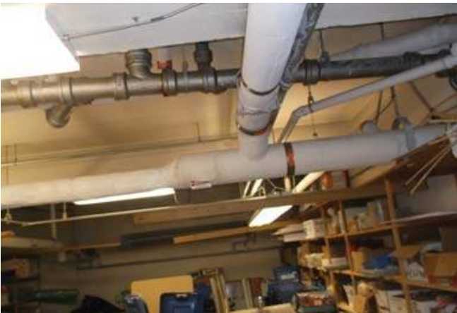
Original Steam Piping with Asbestos Insulation
