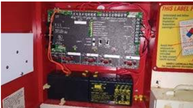
Interior of fire alarm control panel
