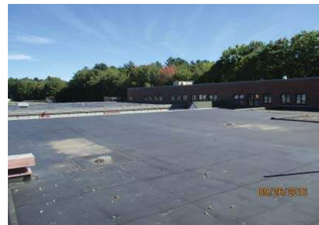
Recommend replacement of roof ballast
