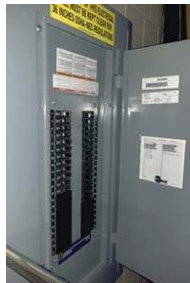
A Recently Installed Branch-Circuit Panelboard
