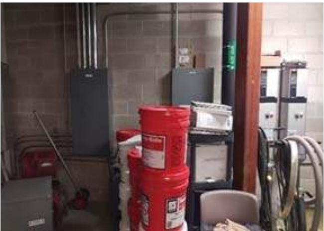
Branch-circuit panelboards
