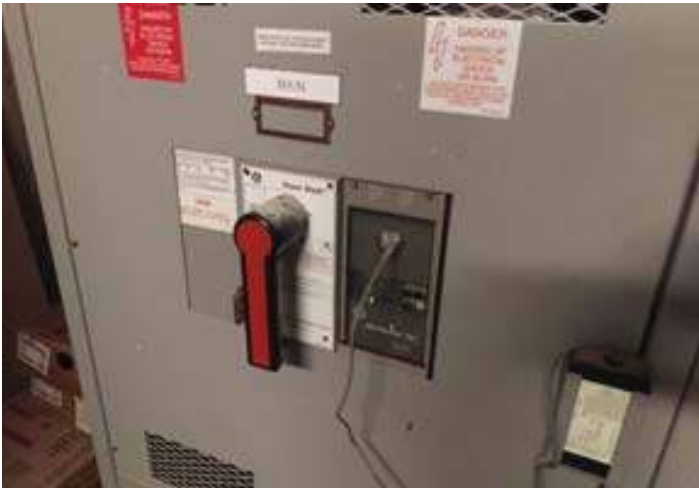
Main circuit breaker at switchboard
