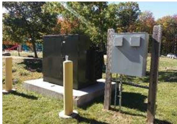
Utility Pad Mount Transformer
