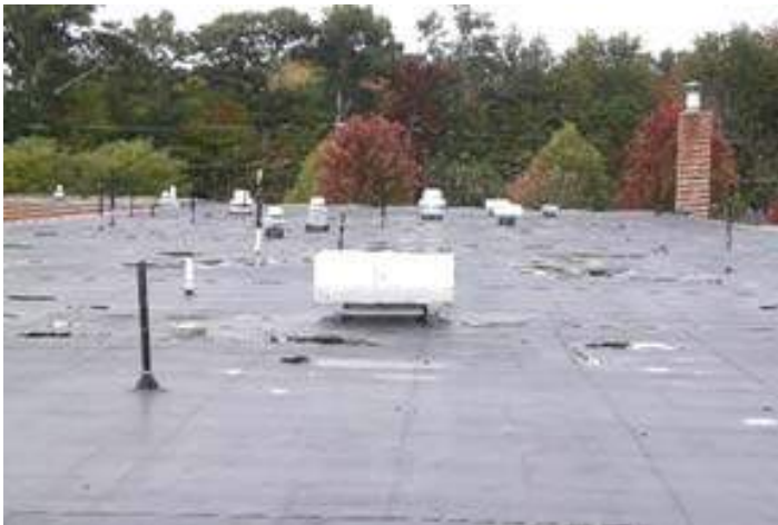
Gravity Relief Ventilator
