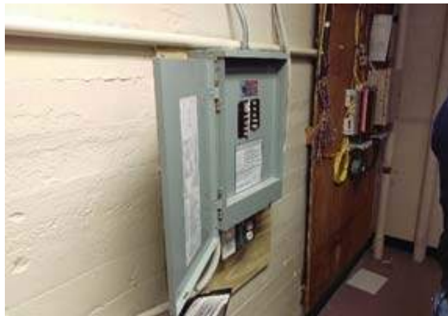
Combination automatic transfer switch/load center
