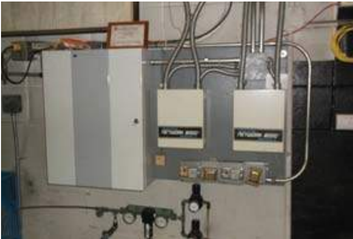
Pneumatic & DDC Temperature Controls
