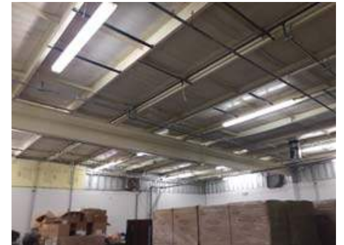
Vapor-tight T8 fluorescent luminaires
