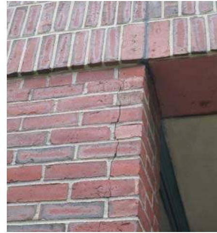
Bearing cracks at long spanning lintels
