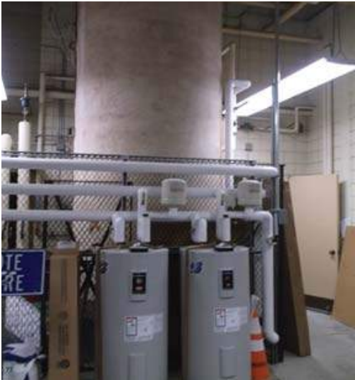
Indirect DWH and storage Addition
