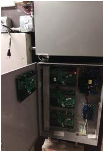
Unused Access Control Panel
