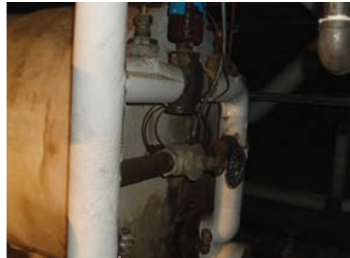
Steam generated DHW & Storage at Gym
