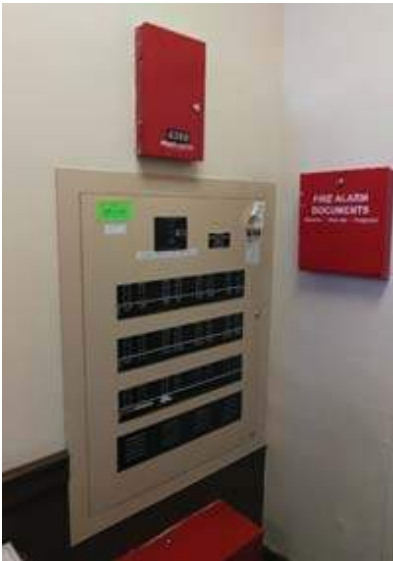
Fire alarm control panel
