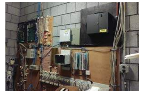
Telephone Utility Demarcation – Much of this equipment appears to be abandoned in place.
