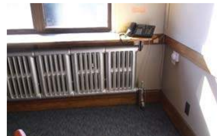
Cast Iron Radiation
