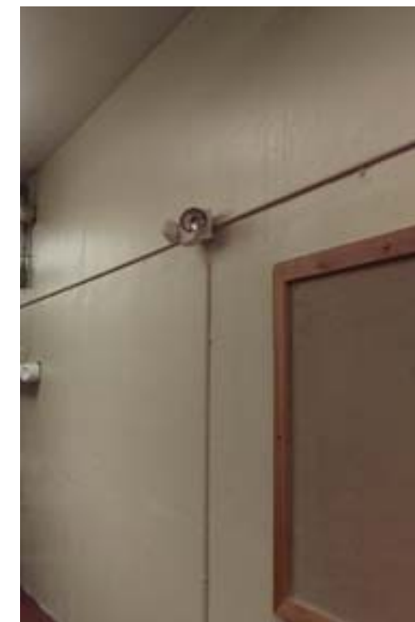
An incandescent emergency lighting unit
