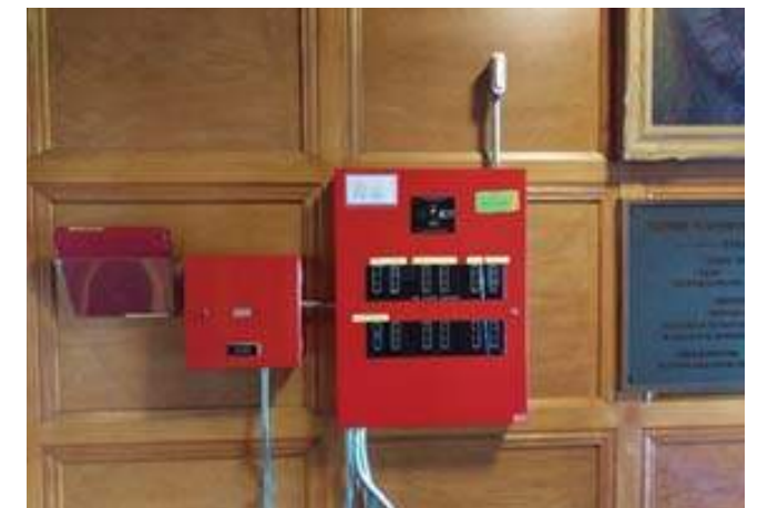
Fire alarm control panel
