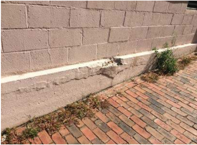
Spalling at foundation
