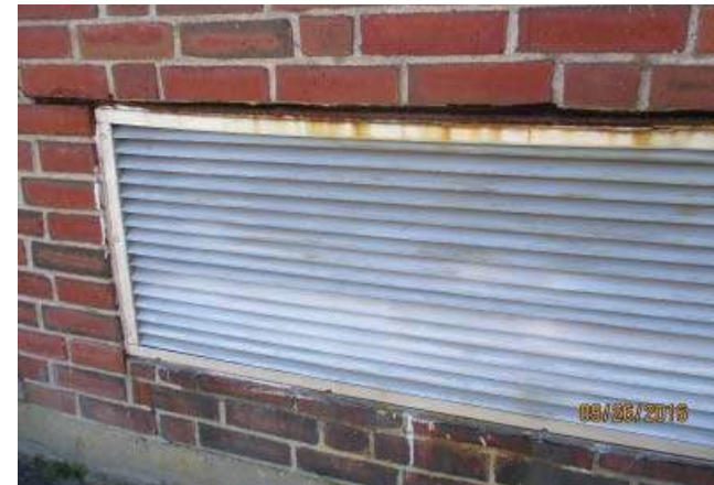
Corroded lintel in need of replacement
