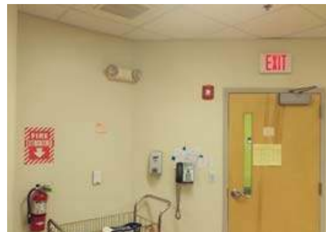
Emergency battery unit with incandescent heads.
