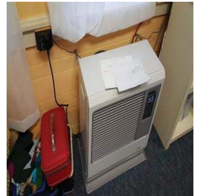
Laser 730 Floor Fuel Fired Heater
