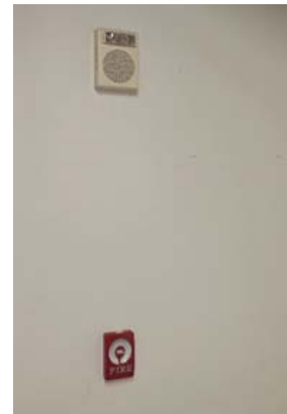
Typical Pull Station and Notification Appliance
