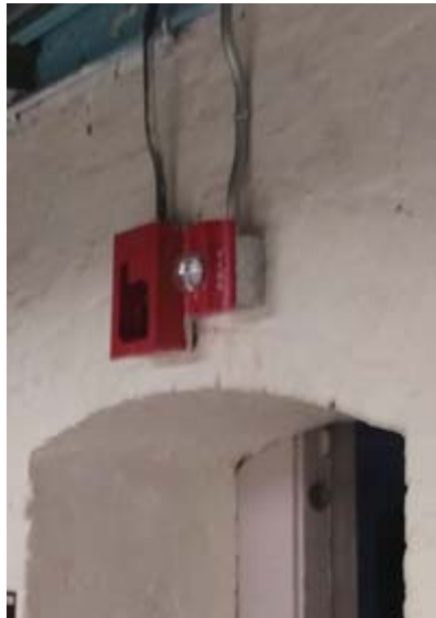
A New Notification Appliance Adjacent to an Old Backbox
