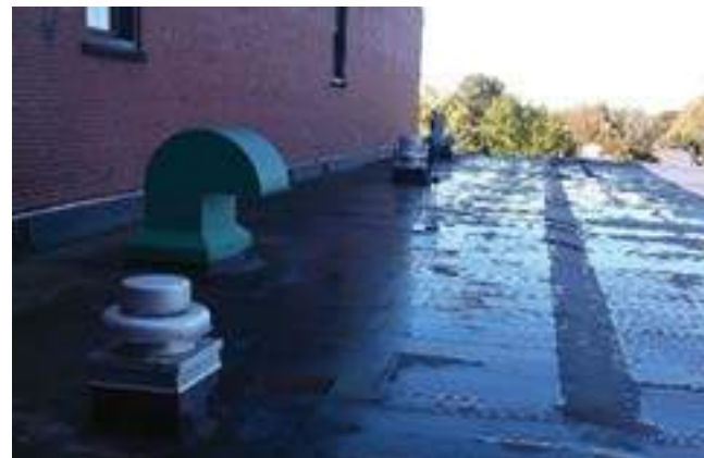
GRVs &amp; Exhaust Fans
