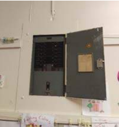
Any old circuit breaker panel – a plastic cover has been field fabricated to cover live parts within.
