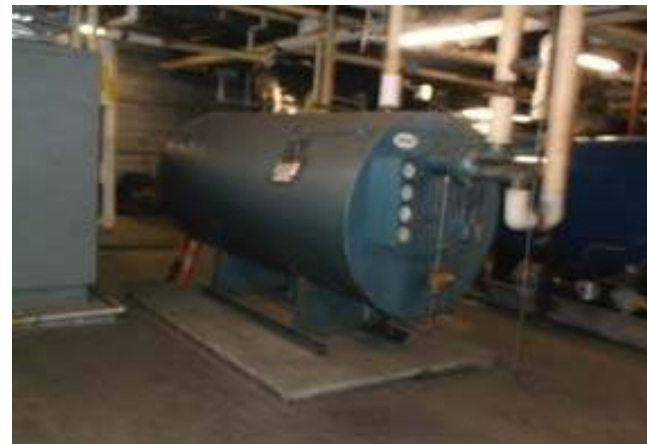
Indirect DHW Heater/Storage
