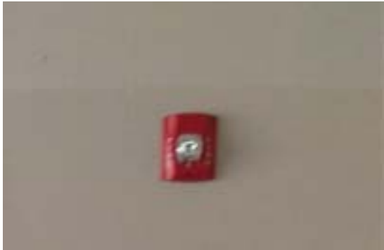
An ADA compliant notification appliance
