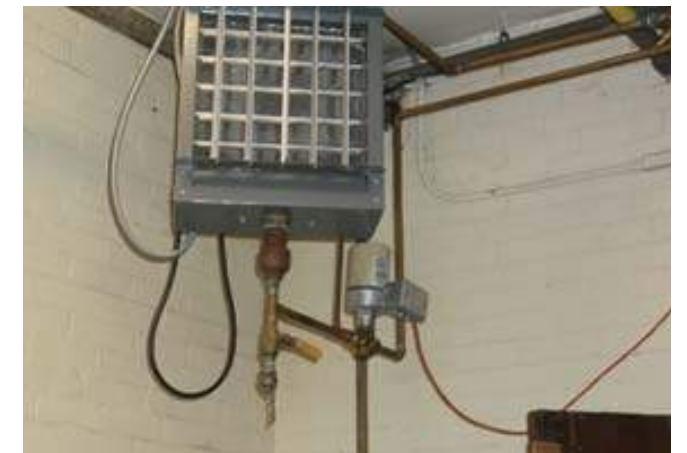
Unit Heater with Hydraulic Valve Actuator
