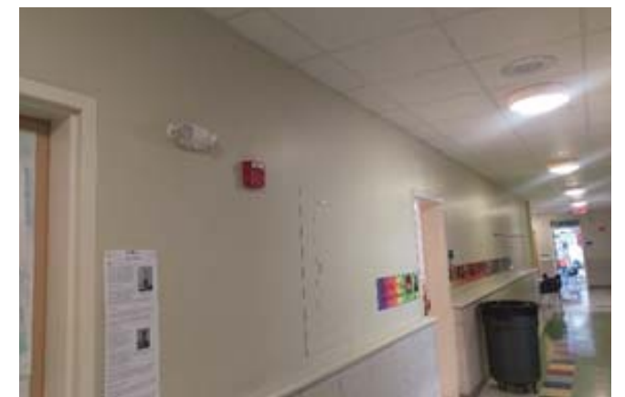
Fire alarm notification in corridor
