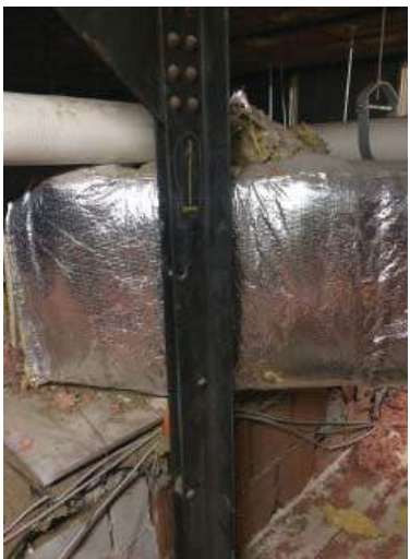
Missing rivet
