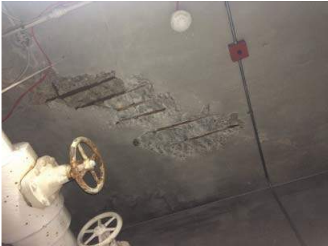
Concrete spalling
