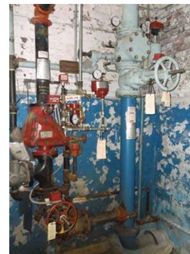
Fire Sprinkler Entrance – Dry Pipe Left Riser
