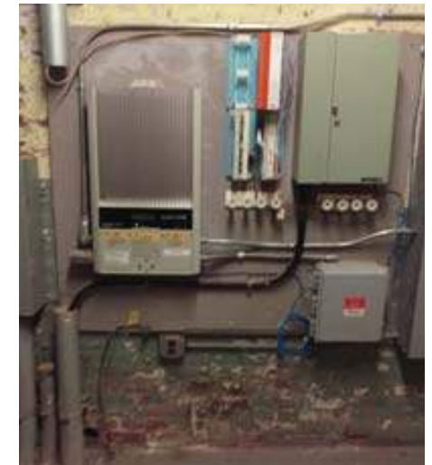
Telecommunications utility demarcation point
