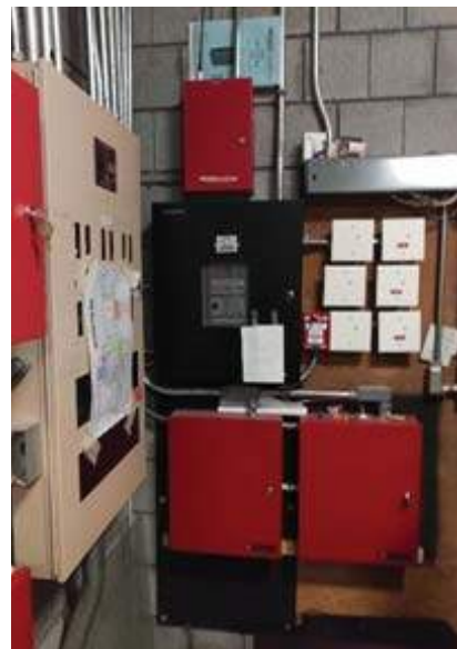
Fire alarm Control Panel and Power Supplies
