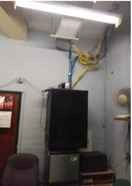
IDF in enclosed rack in shared space
