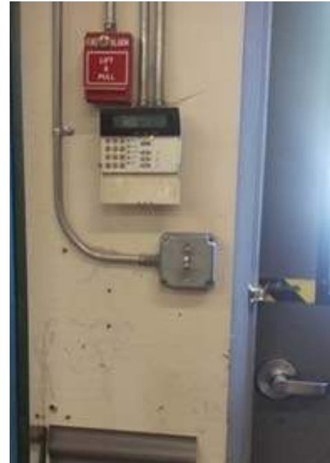
An Intrusion Alarm Keypad
