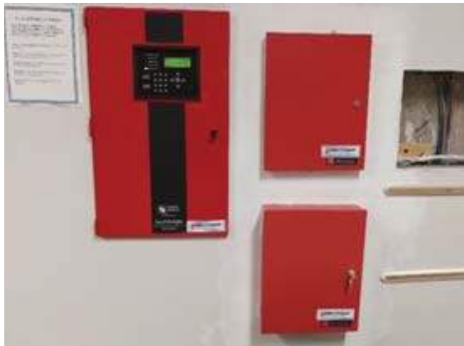
Fire Alarm Control Panel
