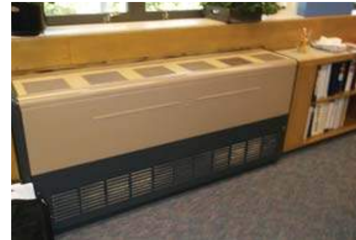
Typical Classroom Unit Ventilator
