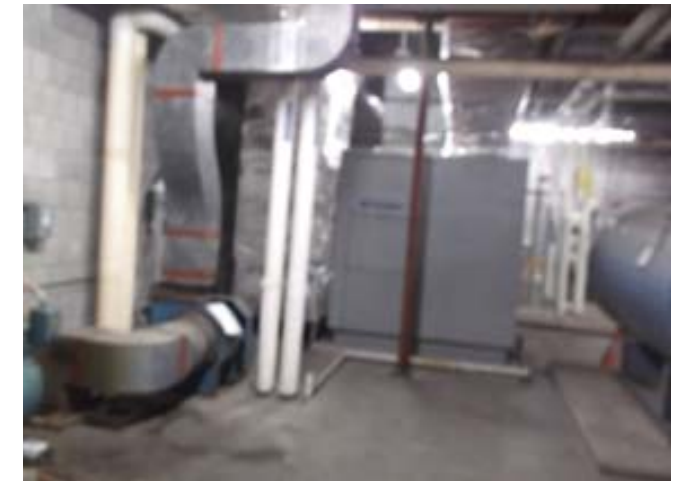
Pool Dehumidification Unit
