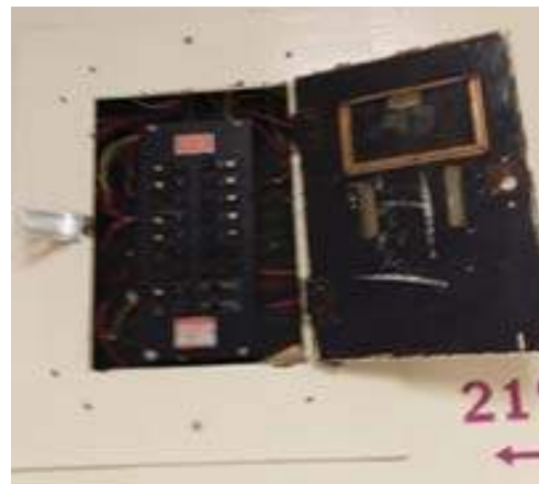
An obsolete panelboard. Most of these have been replaced, but a couple remain
