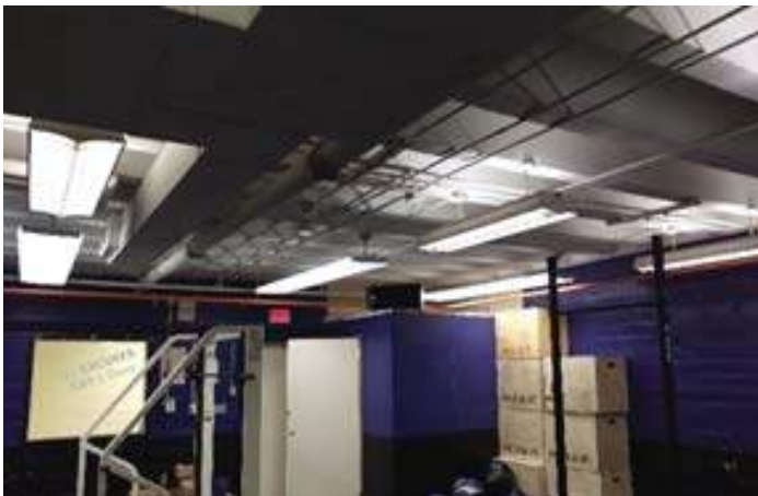
Obsolete louvered fixtures in fitness room
