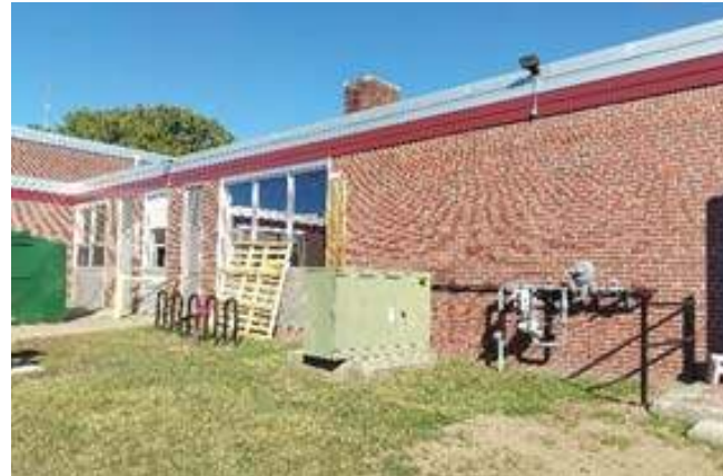
Utility Pad Mount Transformer
