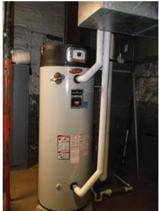
Gas Fired Water Heater
