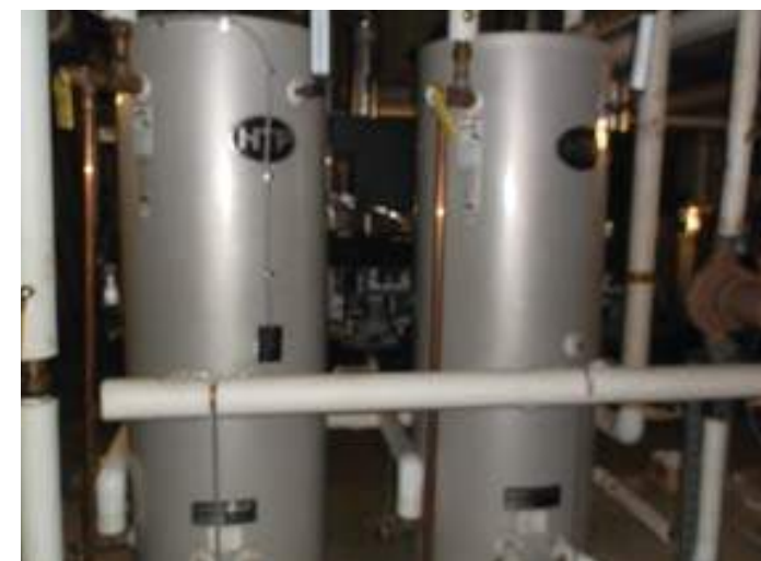
Indirect Water/Storage Heaters
