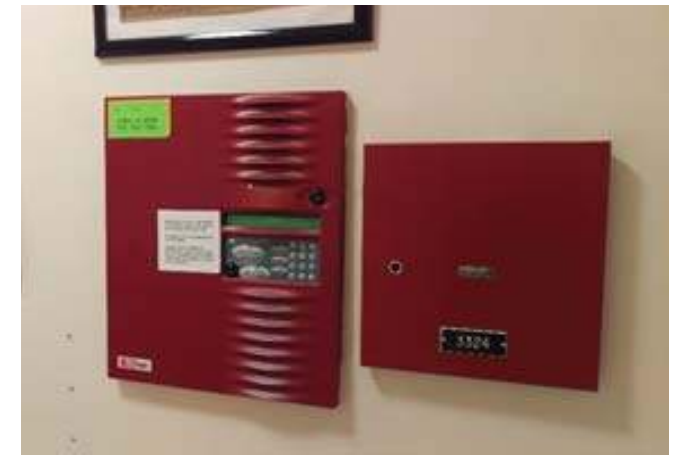
Fire alarm control panel
