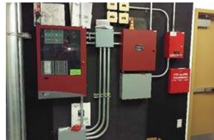
Fire Alarm Control Panel
