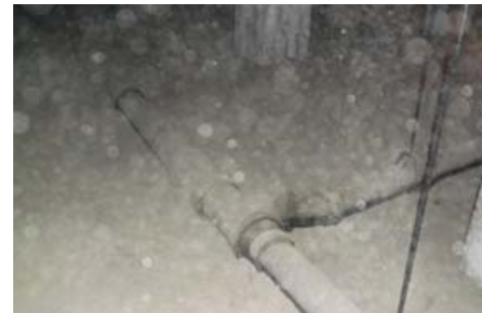
Cast Iron Rain Water Piping
