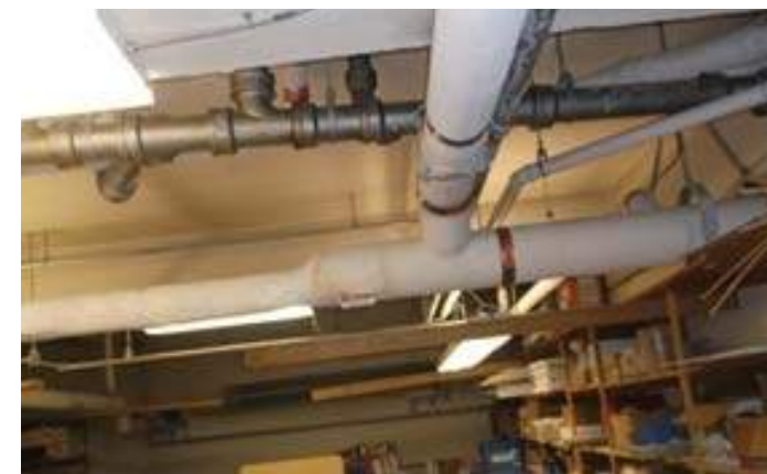
Cast Iron Sanitary Piping
