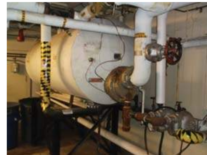
Indirect Steam DWH and Storage Original Bldg
