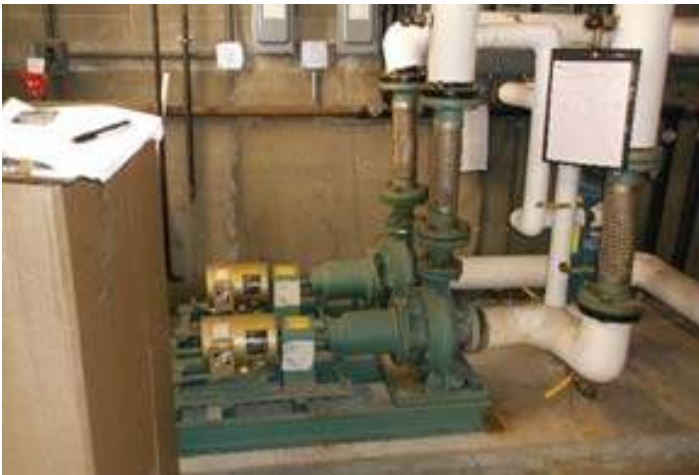
Base Mount Heating Pumps
