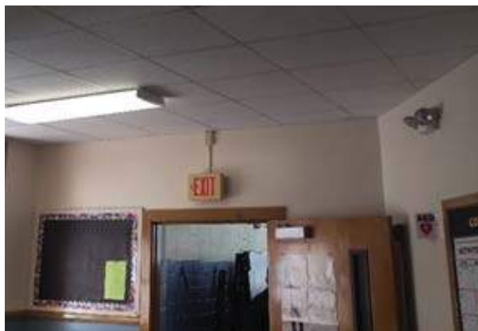
An Exit Sign and Newer Emergency Lighting Unit
