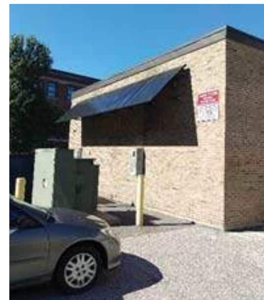
Padmount transformer and PV array
