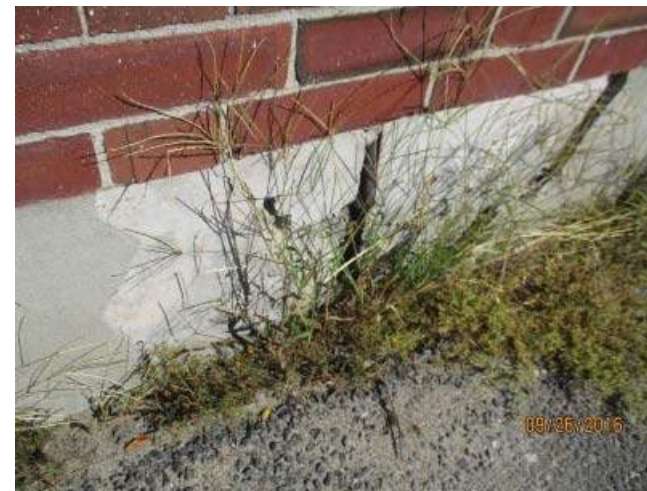
Foundation wall sealant to be replaced
