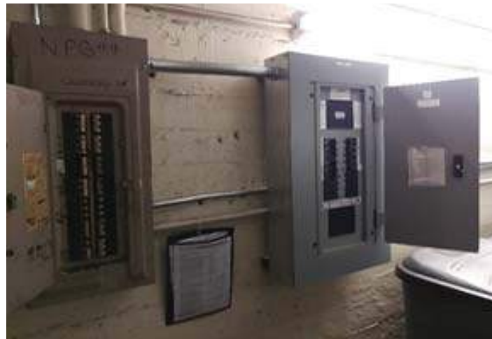
A new panelboard adjacent to an old load center in boiler room.
