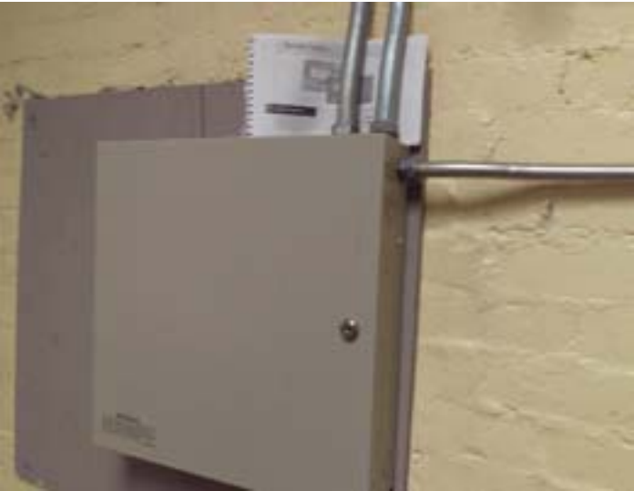
Security alarm control panel
