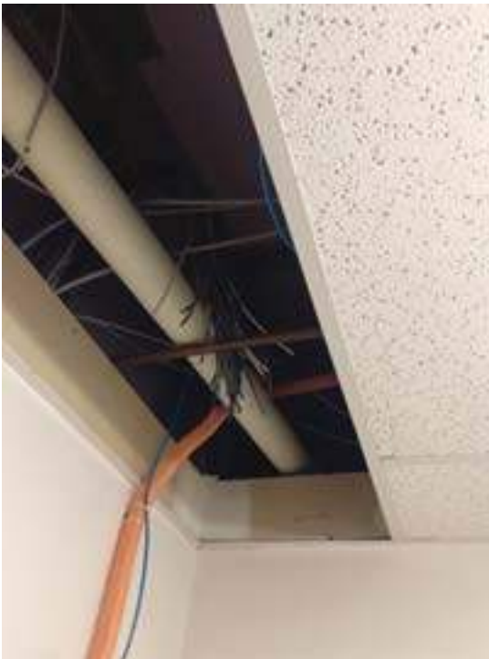
Abandoned cables in First floor IDF room
