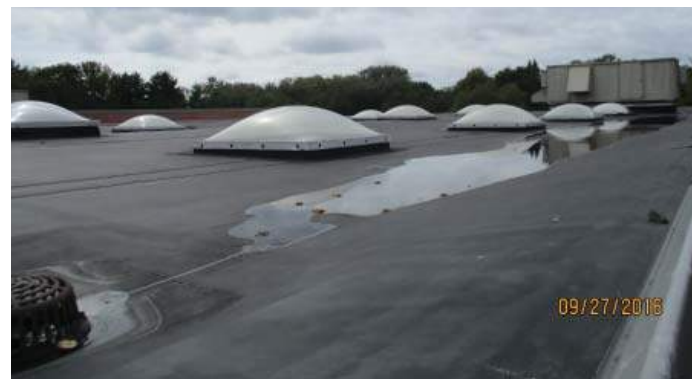
Inadequate roof drainage at Cafeteria roof
