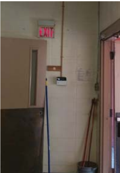
An LED Combination Exit/Emergency Light
