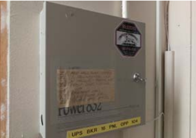
Security alarm control panel
