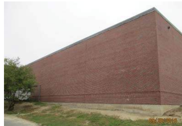
Possible loss of foundation protection at Gym
