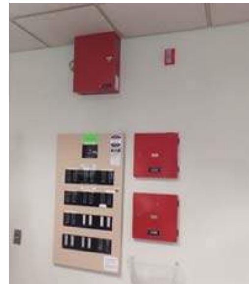
Fire Alarm Control Panel and an Obsolete Strobe
