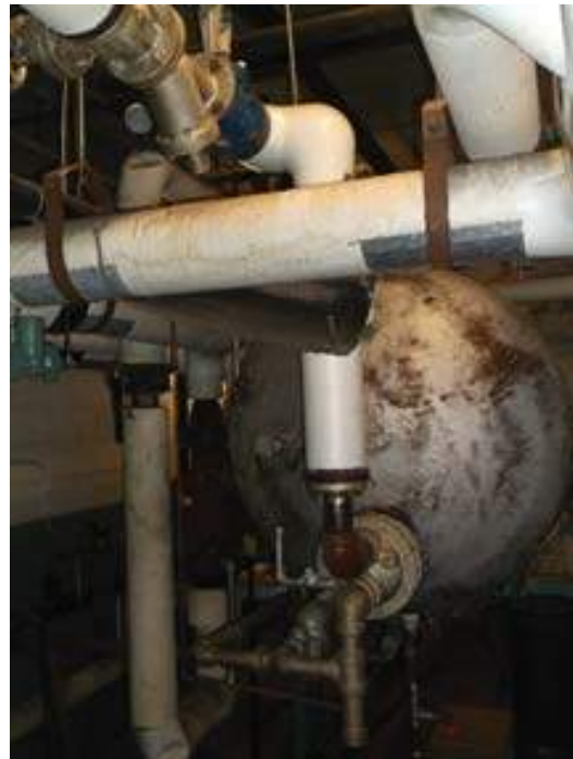
Steam generated DHW &amp; Storage at Gym
