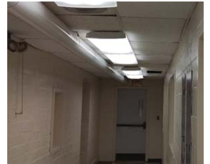
Incandescent emergency light heads and non-illuminated exit sign
