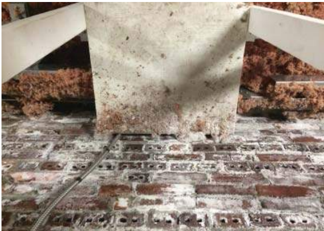
Efflorescence
