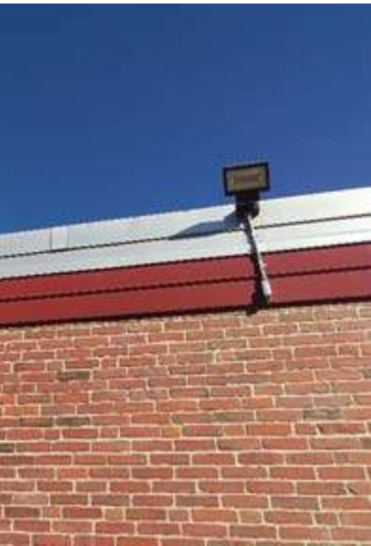
A Typical LED Wall Pack
