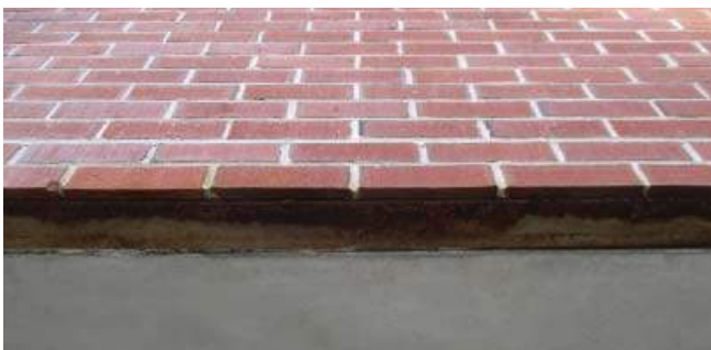
Corroding relieving angle
