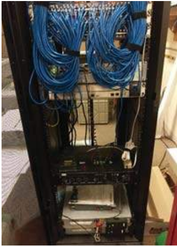
Main Distribution Frame (MDF) with Paging Amplifier
