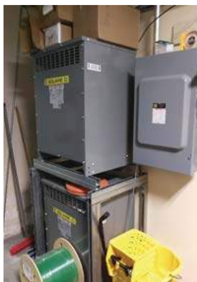
Transformer Installation in Progress in Addition
