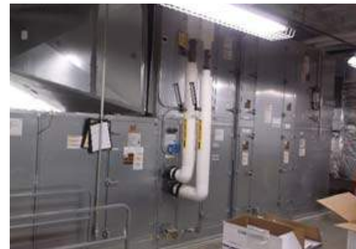
Air Handler Heating Only—Displacement Ventilation
