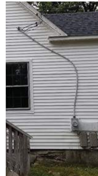
Service entrance and meter enclosure
