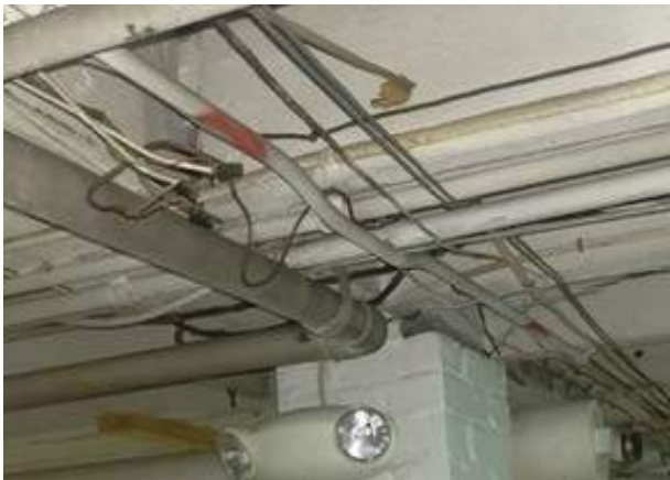
Very Old Branch Circuit Wiring
