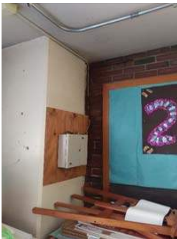
IDF on Second Floor in Shared Space Fiber Optic Termination in a Classroom
