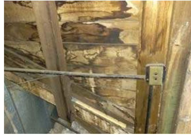
A very old, obsolete light switch in attic. Wiring is presumed to be obsolete cloth-covered conductors.
