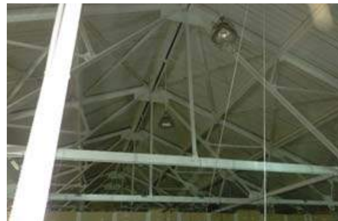
Old lighting and wiring abandoned in attic above old gym
