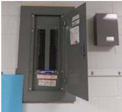
A recently installed Square D panelboard
