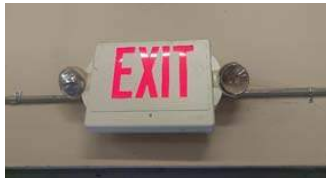
A Combination Exit Sign/Emergency Lighting Unit
