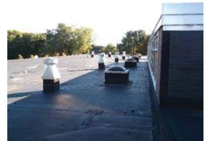
Gravity Relief Ventilators
