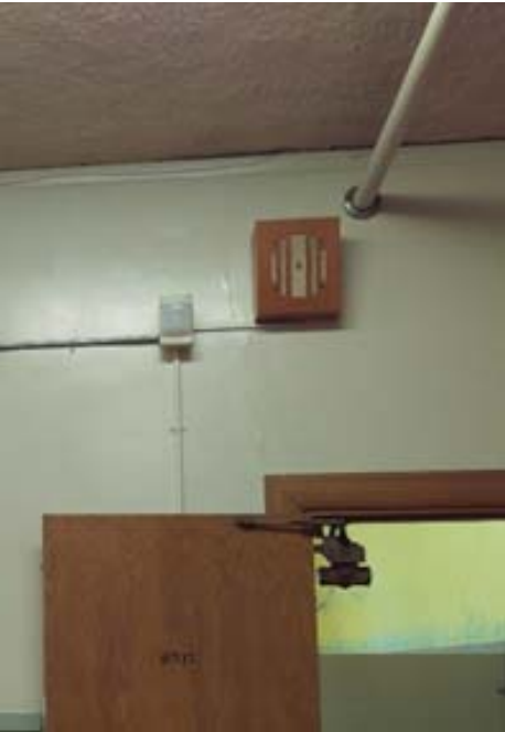
A corridor motion detector
