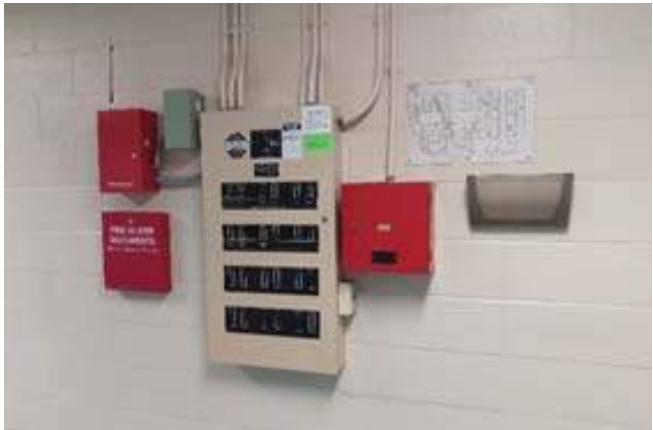
Fire alarm control panel
