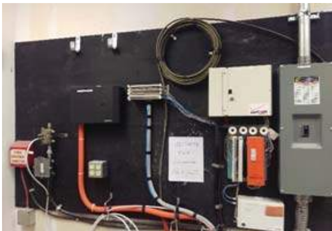
Telecommunications utility demarcation
