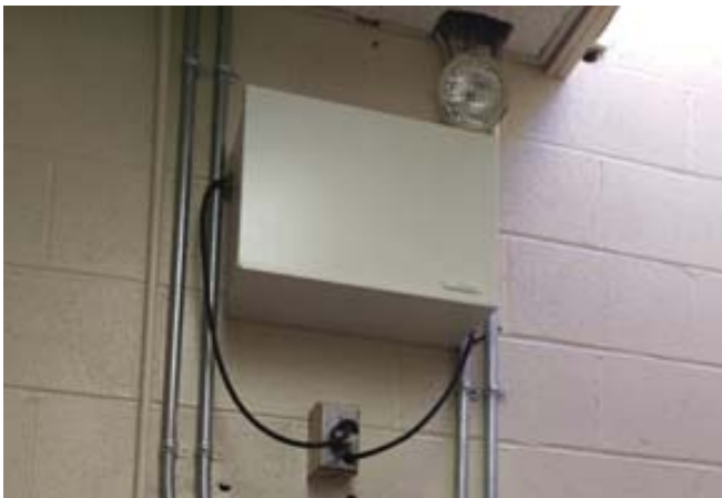
Emergency Lighting Battery Unit
