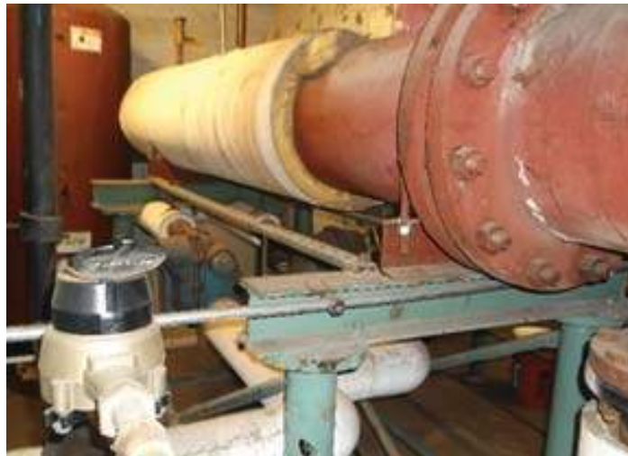
Steam to HW Heat Exchanger
