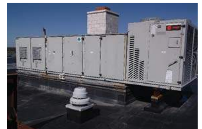
Typical Packaged RTU & Typical Exhaust Fan
