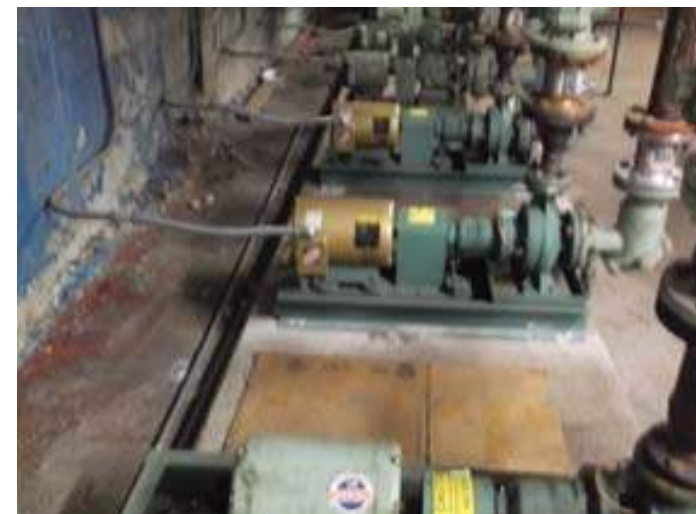
Bank of Base Mounted HW Building Pumps
