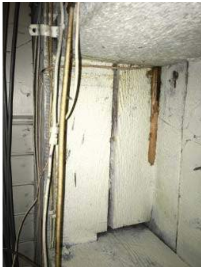
Checked wood in basement
