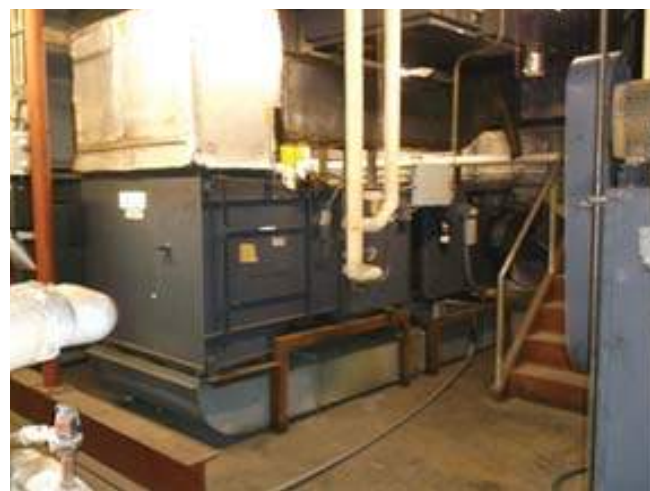
AHU-8 Original Equipment To Be Replaced
