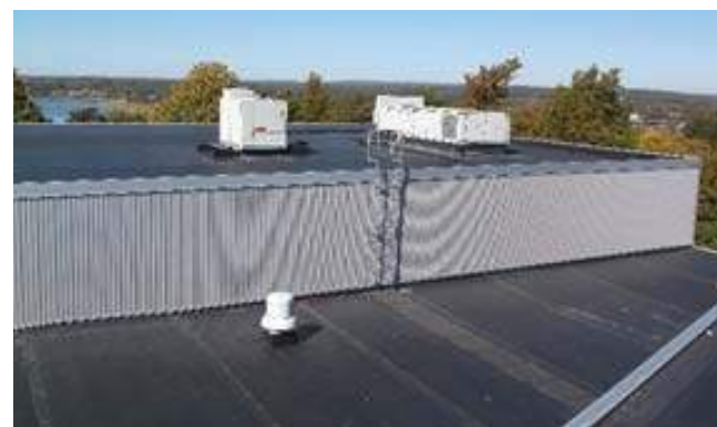
Typical Split DX RTU Serving Gym
