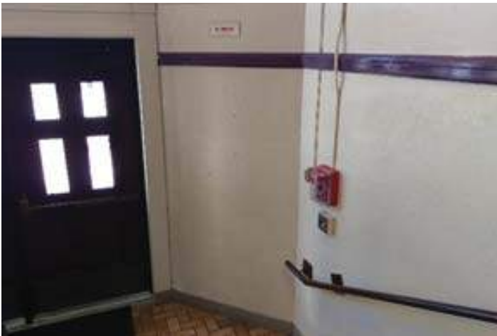
Pull station located too far from exit – a common condition in this building.
