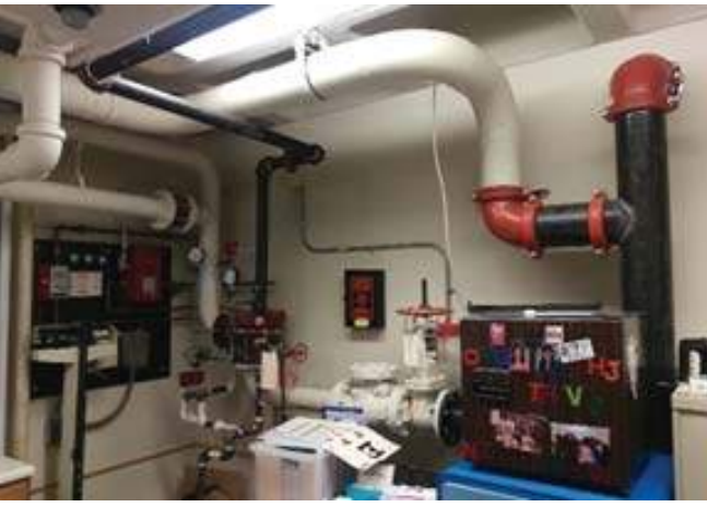
Deluge Control System for Open Resource Area
