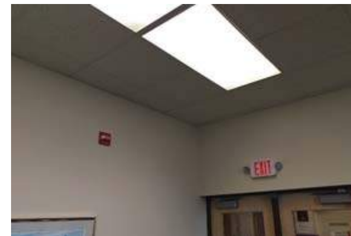
Combination exit sign/emergency lighting unit with integral LED heads
