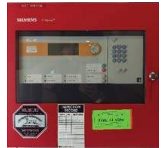
Fire alarm control panel
