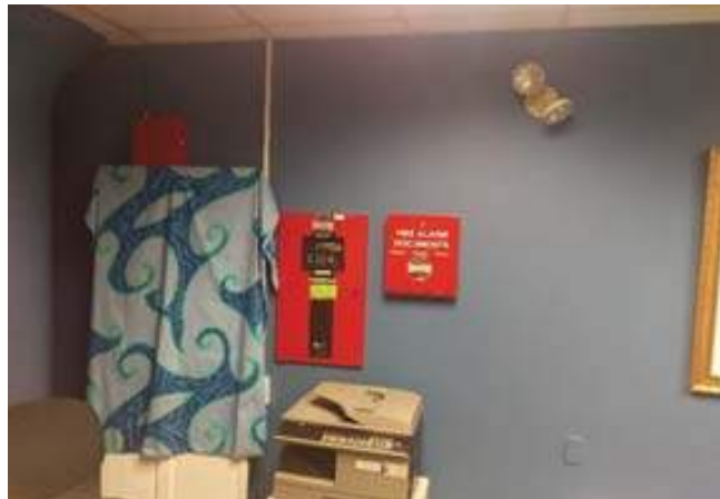
Fire alarm control panel
