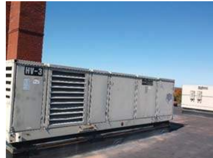
Typical Roof Top H&amp;V unit
