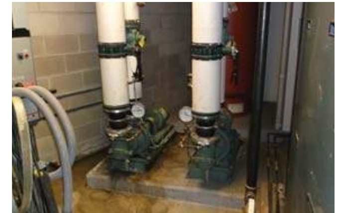
Building Loop Heating Pumps
