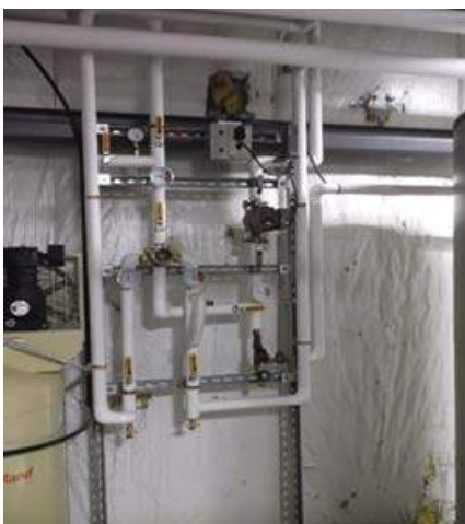
Domestic hot water mixing valve
