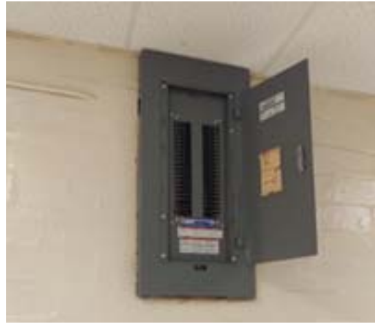
Typical Square D panelboard installed to replace an obsolete panelboard.
