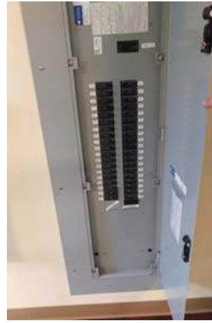
A Typical Branch-Circuit Panelboard
