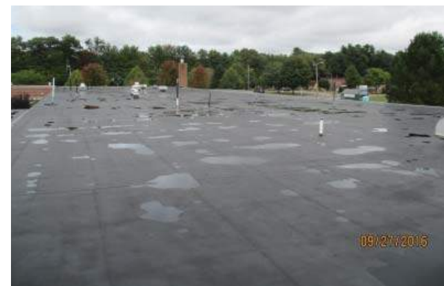
Inadequate roof drainage at classroom addition
