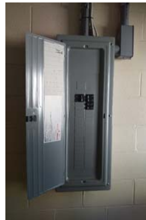
Load Center in Corridor – Feeds Modular Classrooms
