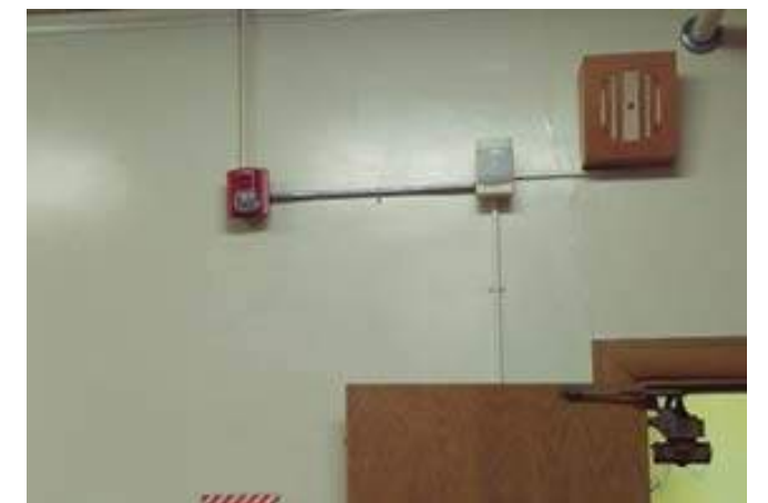
Fire alarm horn/strobe unit
