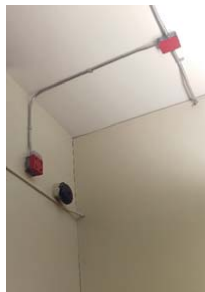
Typical Horn/Strobe Unit
