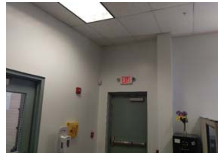
Combination Exit sign/emergency lighting unit
