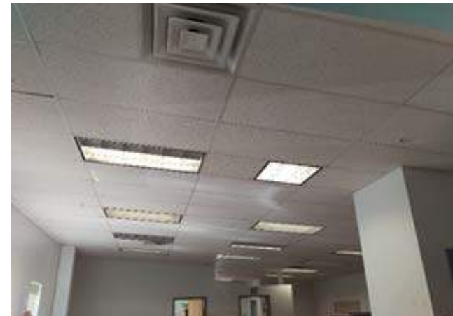
Parabolic lighting in office area
