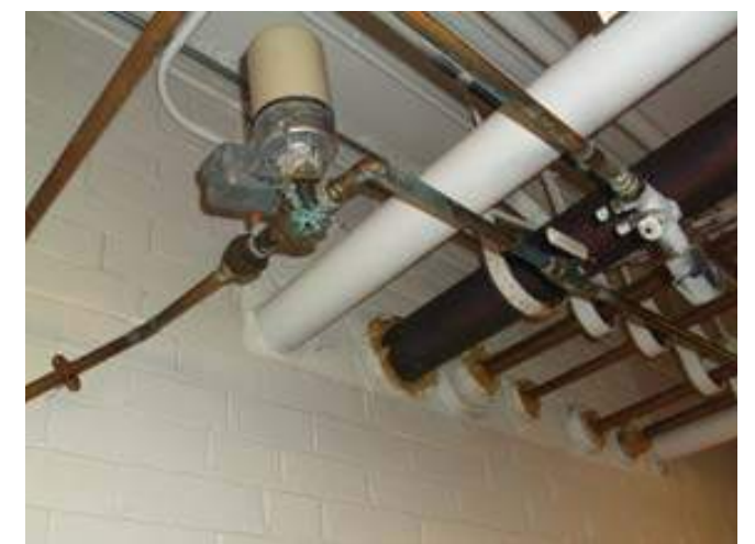
Leaking Actuator and Corroding Solder Joints
