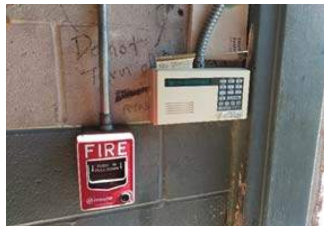
Intrusion alarm keypad
