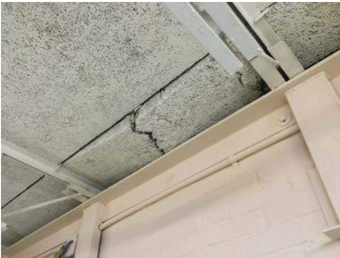
Broken tectum planks
