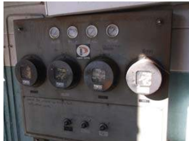
Original Pneumatic Temperature Control Panel
