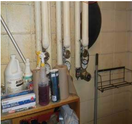
DHW Mixing valves Addition
